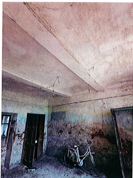
(c) locale al piano terra
